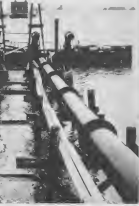
ONCE THE DYKES had been closed the flood waters were returned to the North Sea by means of an extensive network of pipes and powerful pumps. The small vessels in the center hold the pumps that suck water. UNA VEZ e dijknan a worde cerra e awa a worde deshali den Noordzee pa medio di un red extensivo di tubo y pompnan potentes. E barconan chikito den centro ta contene e pompnan cu ta chupa awa di dia y anochi.
